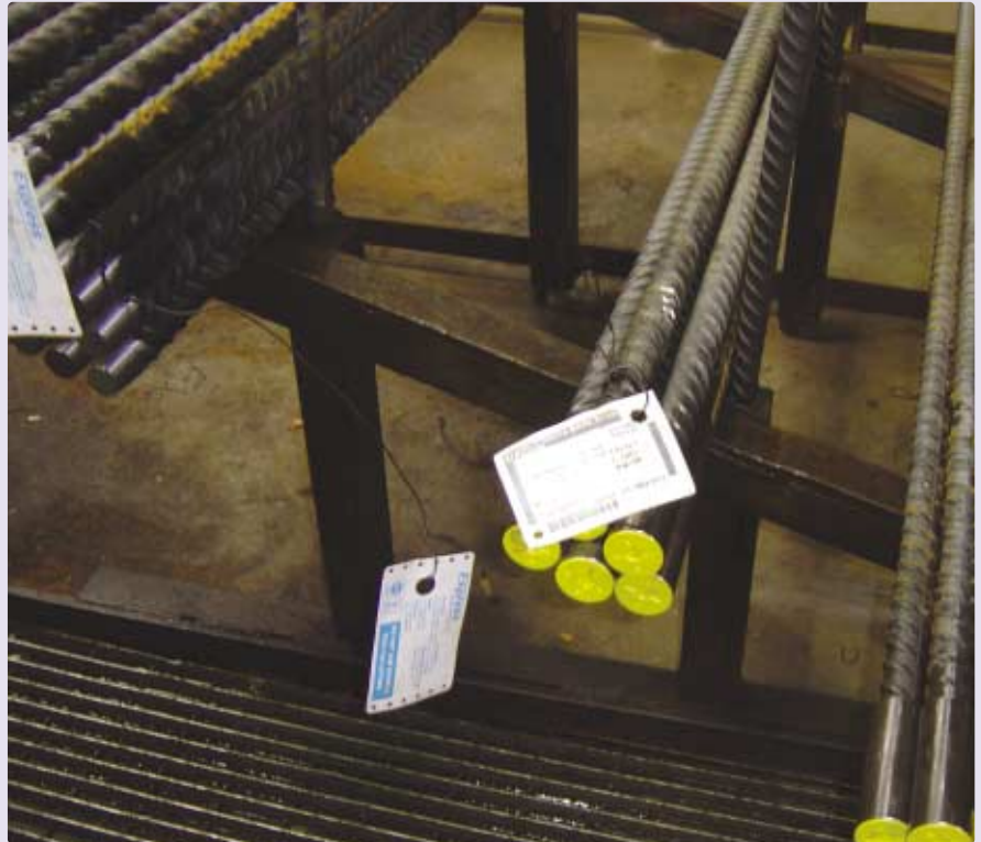
Figure 3 Courtesy of Express O'Rourke JV Ltd
