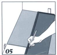
5. At the end of the row, place the last board face down on the floor. the small side with the tongue against the wall. Provide a space of 8mm and transfer the cubing profile to the board.
