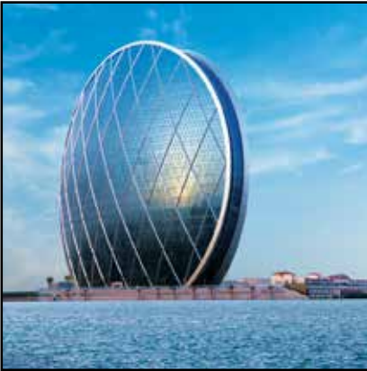
ALDAR HQ Abu Dhabi
