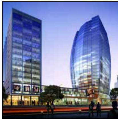
PORT BAKU TOWER Baku
