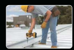
Fixing Screws on Roof
