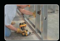
Fixing Structure for Drywall Installation
