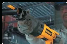
Cutting Pipe Sections to Make Joints
