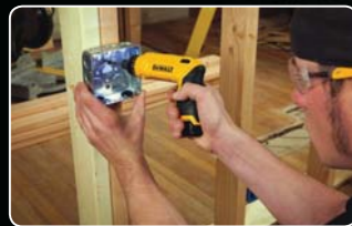
Electrical Fittings on Wood
