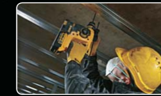
Drilling Holes in Ceiling For Dry wall Installation
