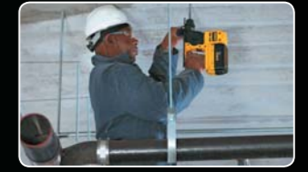
Drilling Anchor Holes in Ceiling For MEP Applications
