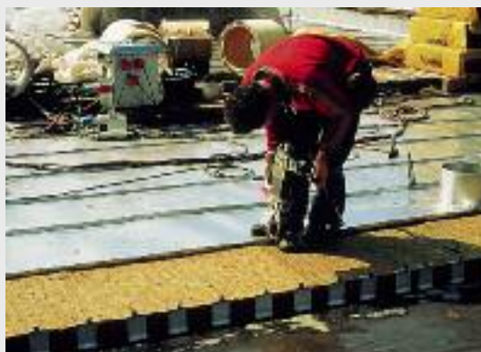
In the warm roof with e.g. mineral fibres or rigid plastic foam, fastening is done mechanically between the metal covering and the load-bearing shell. The result: thermal bridges! In addition there is the question: How secure is the vapour/air barrier?
