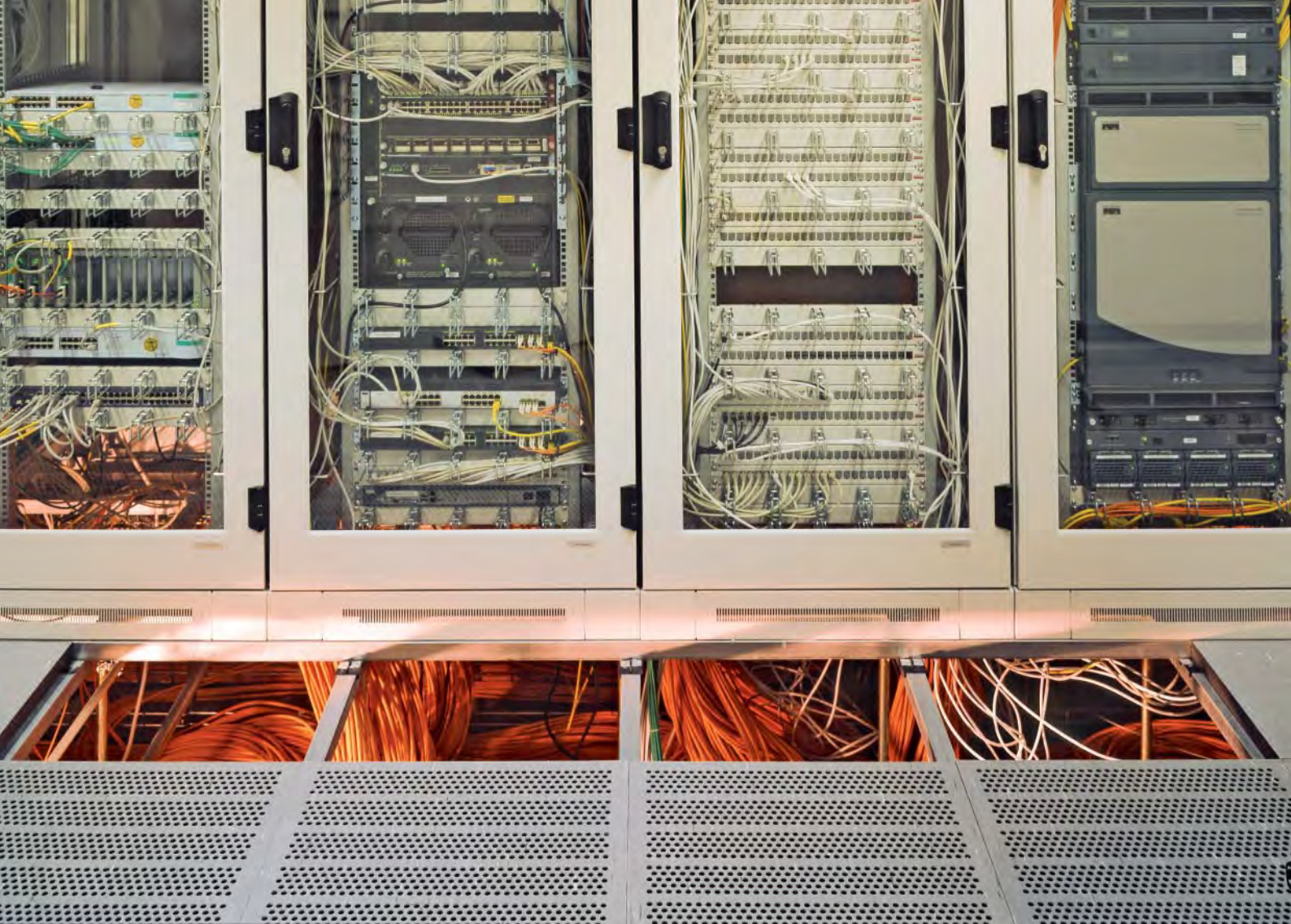
Power Station, Unterföhring
