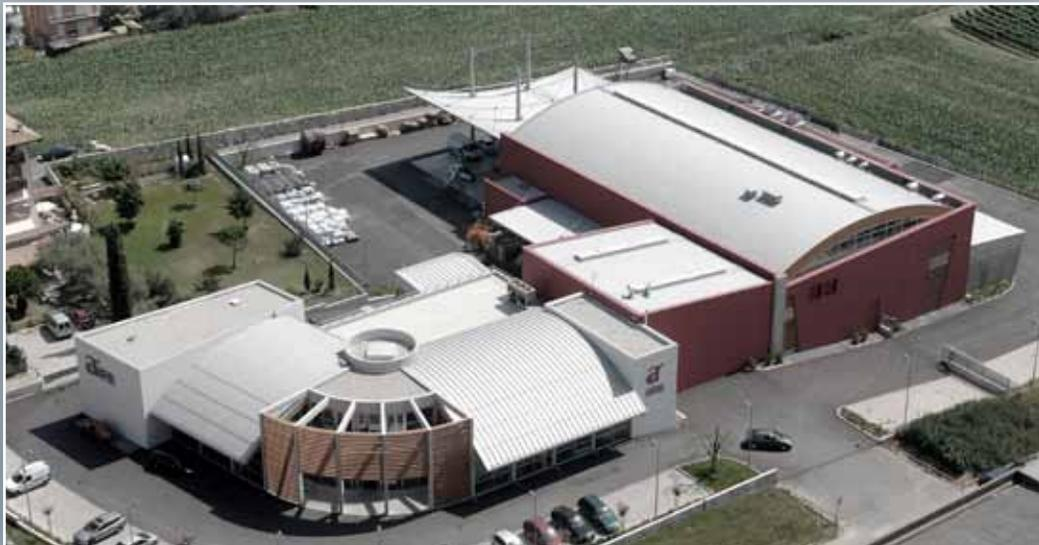
TSSC offers one of its kind and unique roofing system, the seamless flat roof metal covering system where the sheets are joined together using the snap lock system. The latest offering from TSSC is used in industrial as well as in civil building and complies with the latest architectural trends. With its essential shape, aesthetic appearance, constructive economies and outstanding technical properties, seamless roofing system is the perfect balance between technology and appearance
