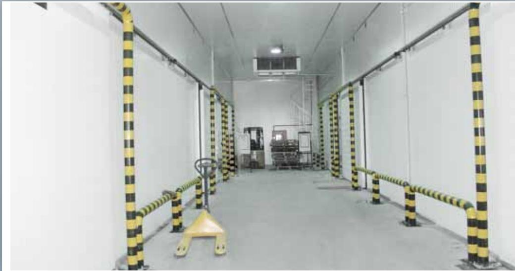
Depending on the size and use of the cold room, cold rooms can be broadly classified as walk-in cold rooms and warehouse cold stores. Cold rooms are built by TSSC to maintain a temperature range of 15°C to -40°C. Walk-in cold rooms are smaller in size compared to the large warehouse cold stores and are used primarily by the retail industry to store goods with fast shelf replenishment rate.
