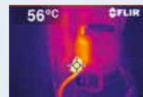
What a thermal imaging camera sees
