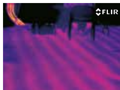
Leaks in an underground district heating network.
