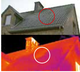
The thermal inspection locates missing insulation in the roof. This can now be repaired and further energy loss prevented.
