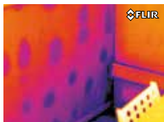
The thermal image shows mould on the interior wall due to water infiltration.
