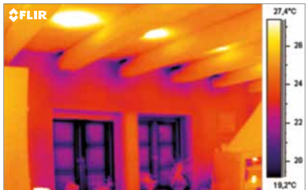
The thermal image shows thermal bridges between the roof beams and adjacent walls.
