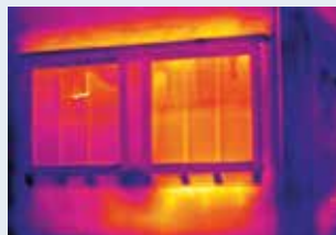
What a thermal imaging camera sees.
