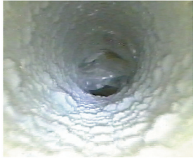
Dirty supply air duct in a hospital
