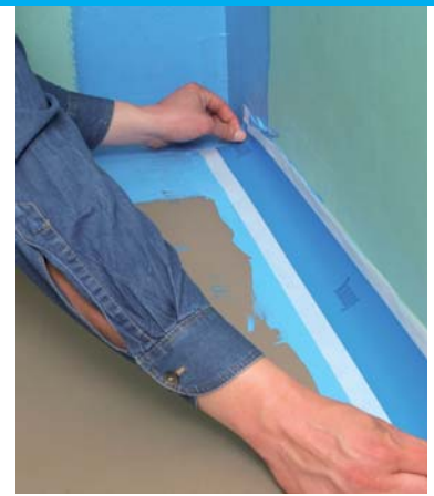
In case of wall/wall and floor/wall junctions Knauf Waterproofing Tape is applied the same way.
