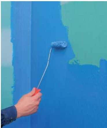
Apply undiluted Knauf Waterproofing to the substrate as a first protective coating to cover the entire surface.
