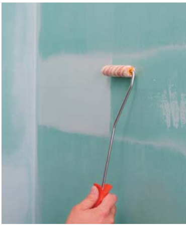
Priming absorbent mineral or gypsum-based substrates and plaster boards with Knauf Primer
