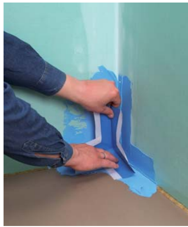
In corner areas Knauf Waterproofing Corner is embedded in a fresh applied coating of Knauf Waterproofing. Pipe connection are sealed with Knauf Pipe-Lead-in Gaskets.
