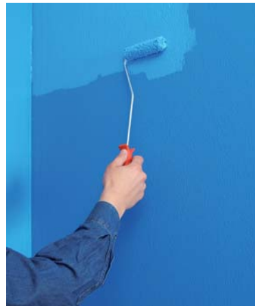
After complete curing of the first coating (approx. 6h) a second coating of Knauf Waterproofing is necessary.
