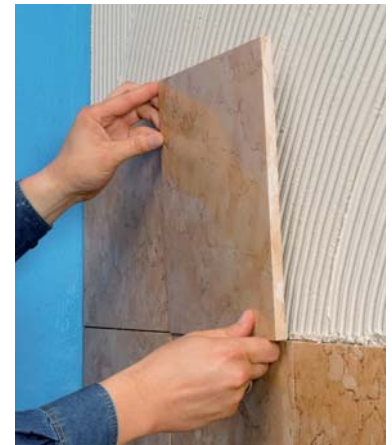
When the second coating of Knauf Waterproofing has cured completely, tiles and stones can be installed.
