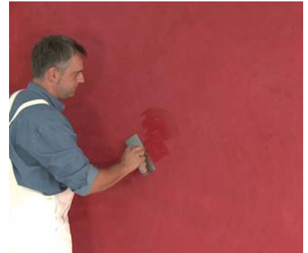
After drying the first layer apply the second layer the same way until the desired gloss level is reached.
