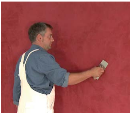
Remove dust and polish to a high gloss with the Venetian smoothing trowel.
