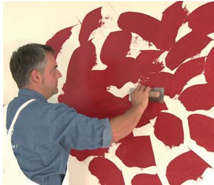
Apply the first layer of Knauf Stucco Design with Venetian smoothing trowel (crossways) thinly.
