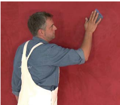
Then dry sand down by hand with P1200 grit sandpaper.
