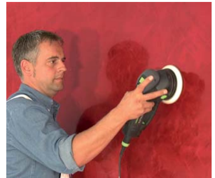
Alternative: manually sand down with P1200, remove dust and finally sand down using P2000 with the Rotex RO 150 FEQ of Festool.
