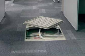
Calyon Bank - Regional Head Office DIFC, Dubai, United Arab Emirates 700 m2 This project used the CF Series panels with bare finishes on T3 pedestals with a finished floor beight of 150 mm
