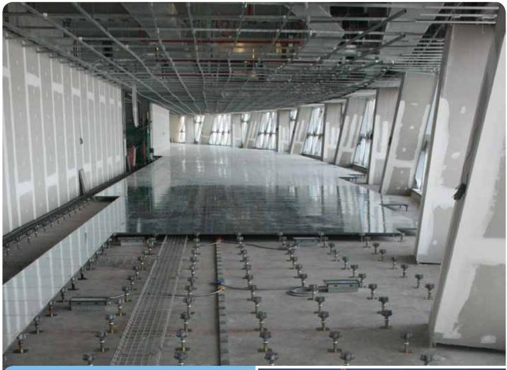
ALDAR Properties Headquarters Abu Dhabi, United Arab Emirates 55,000 m2 This project used the WF series galvanized finish panels with T3 pedestals. The finished floor beight is 150mm
