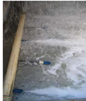
A complete LAKOS basin cleaning filtration system includes a centrifugal separator, pump package, and HydroBooster spray nozzles strategically placed in the tower basin to direct the flow of dirt to the separator.
