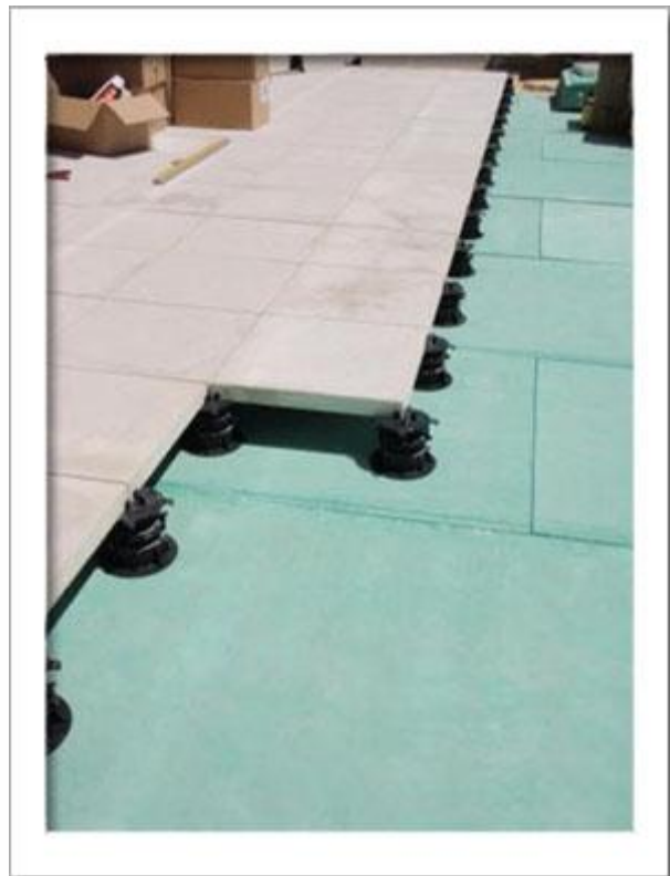
VersiJack ® paver supports positioned on insulation board (above) at the University of Adelaide and part of the completed job (left).
