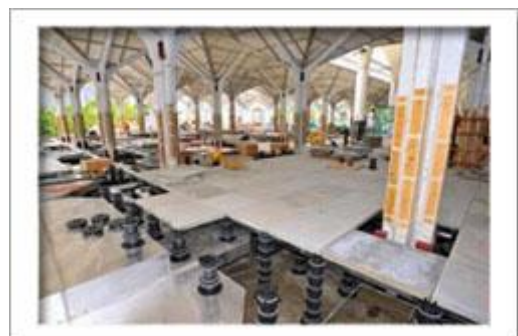
VersiJack ® supports were used in an installation in a mosque in Kuala Lumpur. Each unit supports a load of up to 1.5 tonnes. It also enables easy access to services under the paving.
