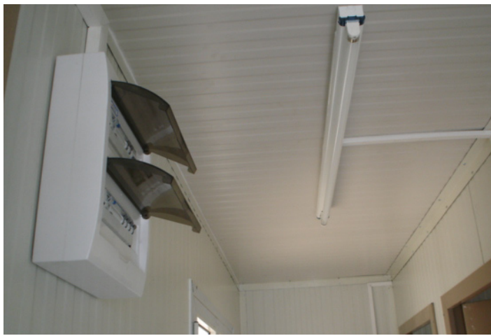
Electrical Distribution Board
