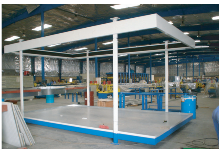
Removal of top frame
