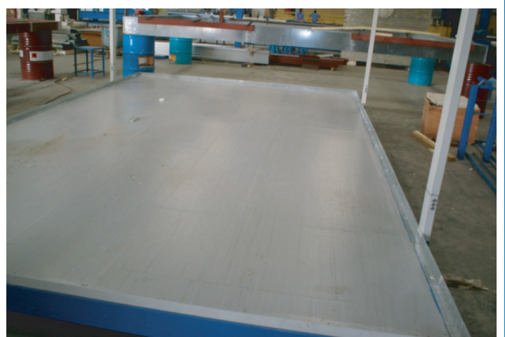
Removal of vinyl flooring
