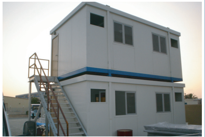
Assembly of bottom and top cabin
