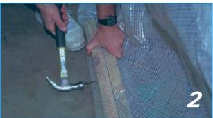
Roll up the excess material with a 1x4 or 2x4 and nail it securely to the pallet.
