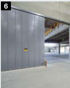
6 Fire sliding doors
