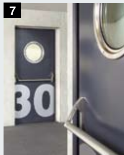
7 Multi-function doors and reinforced internal doors
