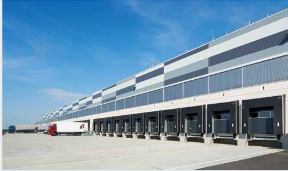
Logistics Operator WA 300 S4 (see page 66), the affordable solution for logistics doors
