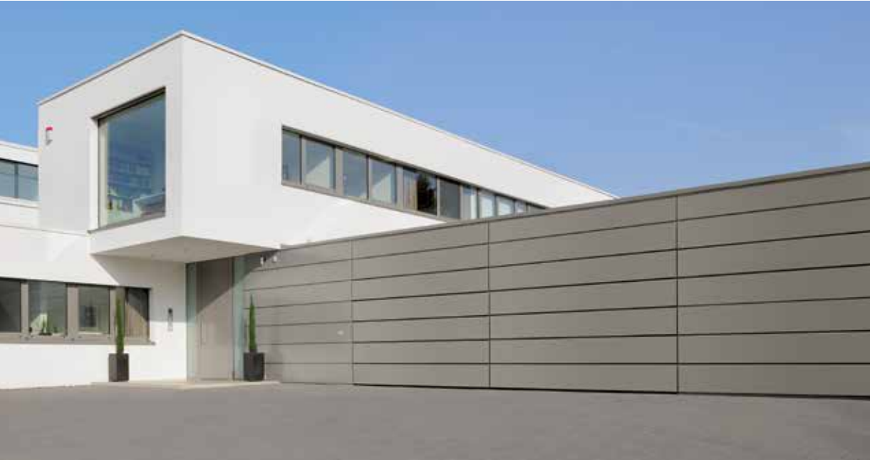
On-site cladding with aluminium compound board
