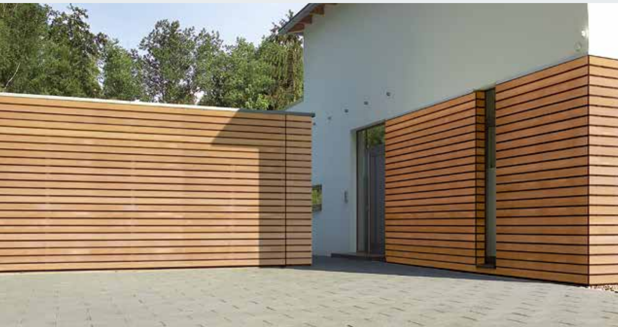
On-site cladding with timber panels
