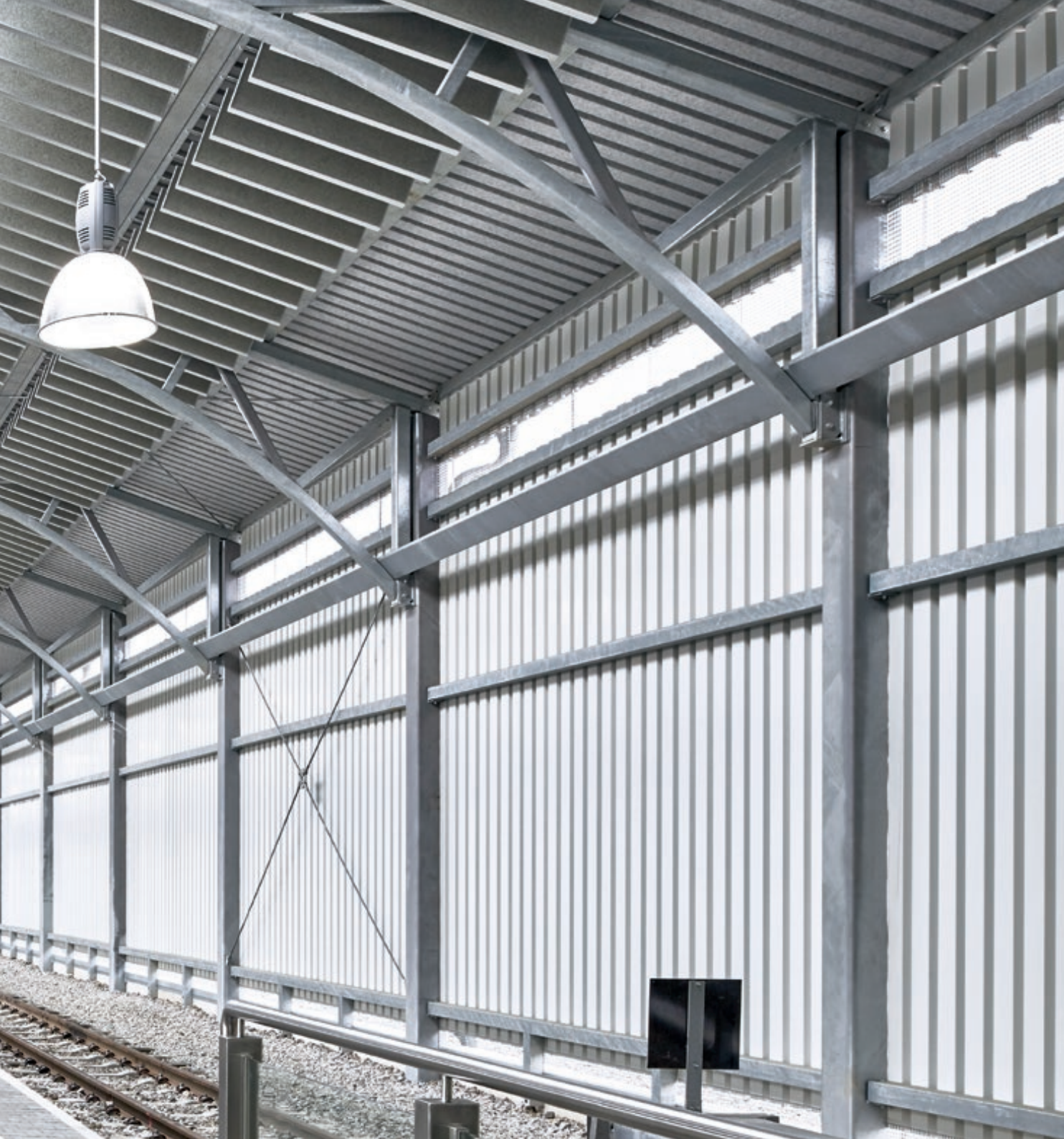
Waldviertelbahn Train Station, Gmünd, Austria, HERADESIGN® Baffle aluDesign superfine A2
