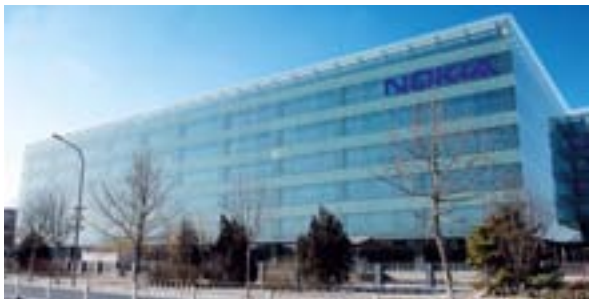
Nokia Headquarters Business Building, Beijing, China
