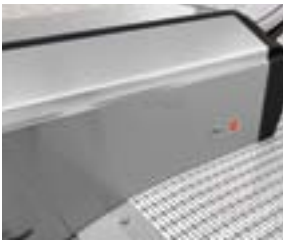
Brushed satin stainless steel skirt with clear anti-friction coating
