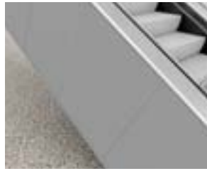
Grey powder coated sheet steel cladding (RAL7036) ***
