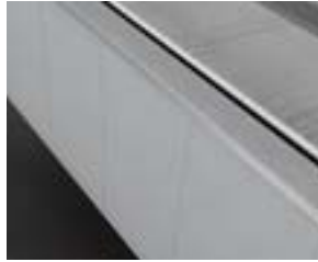
Grey powder coated sheet steel cladding (RAL7036)
