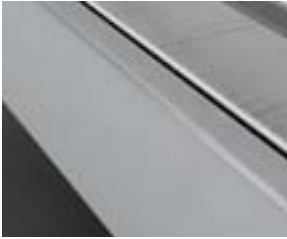
Grey primed sheet steel cladding (RAL7036)
