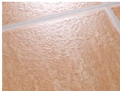
TI (tiles): tile appearance with original joint pattern
