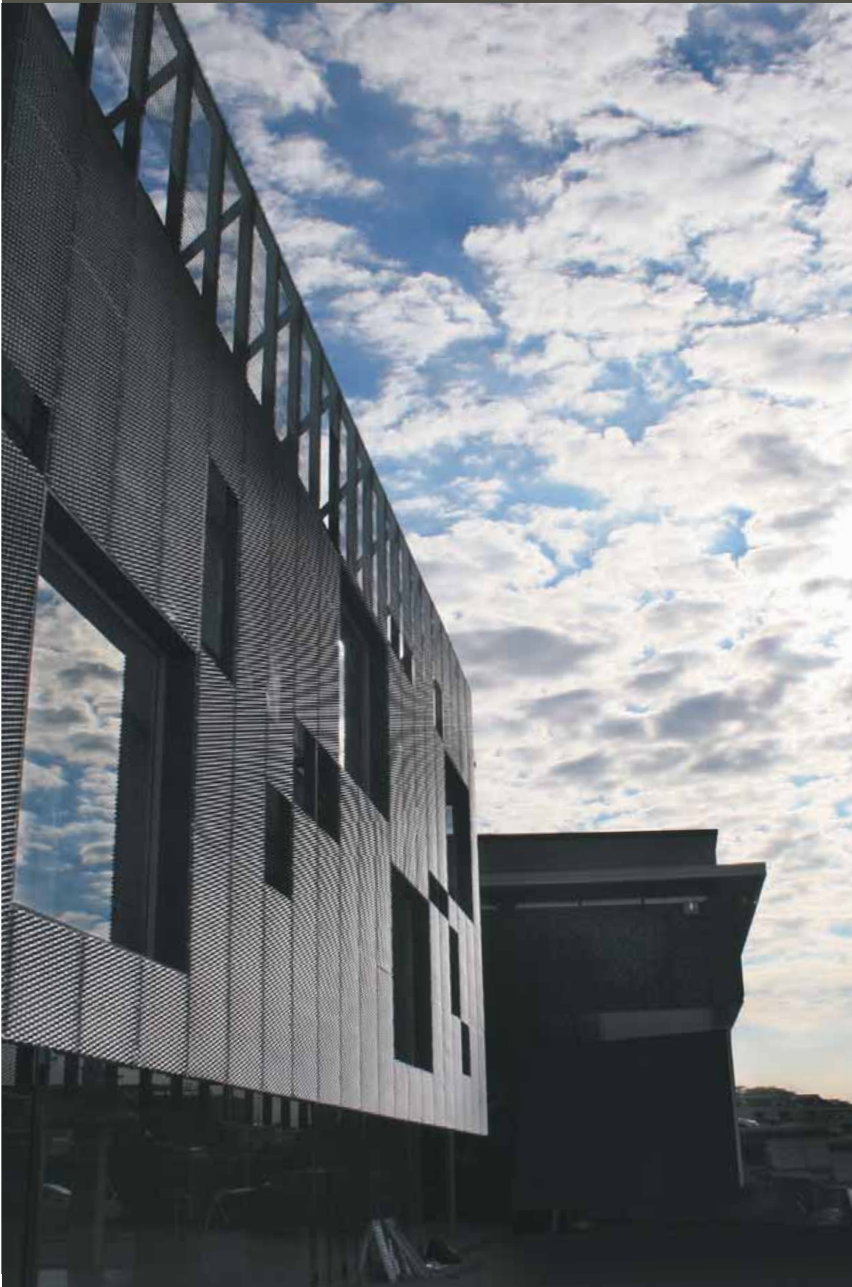
FACCIATA VENTILATA CONCESSIONARIO MOTO TORINO - ITALIA VENTILATED FACADE MOTO DEALER TURIN - ITALY
