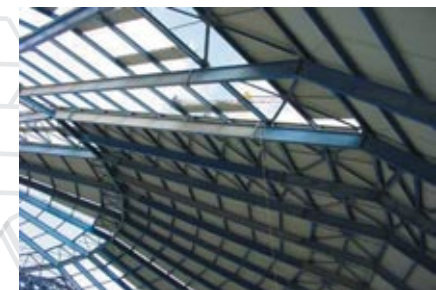
C - purlin on Dome Project
