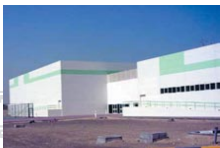
Cold Storage - Iran
