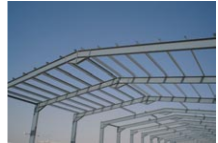
Z - roof purlin on Industrial Shed
