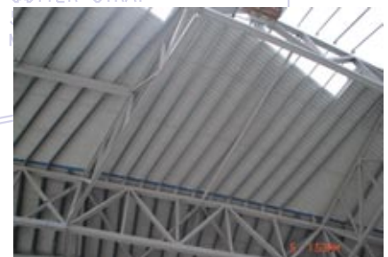
Internal Insulation Envelope at Snow Centre Dubai
