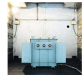
Controllable oil filling under vacuum.
