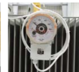
Winding Temperature Indicator
