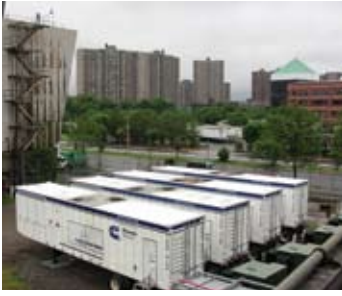
Standby power for a cooperative of 35 high-rise buildings & 7 town-house clusters in New York, USA.
