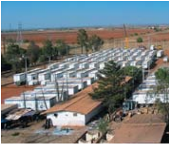
Rental Power units creating emergency power stations at two sites in just 41 days when low water levels in major dams were unable to supply power near Zacatecas, Mexico.
