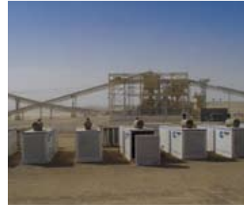
Long-term (10 years) prime power for a gold mining operation in Bulghah, Saudi Arabia.
