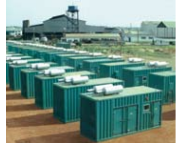
Countrywide replacement prime power when drought caused failing output from a hydro electric dam in Tema, Ghana.
