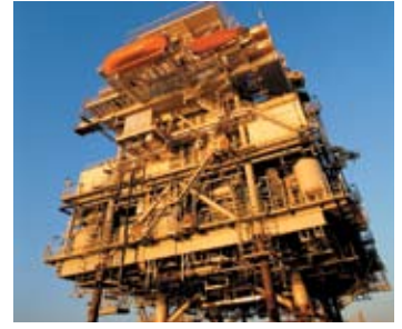
Temporary power station for capacity testing of pumping systems for a deep sea platform off Texas, USA.
