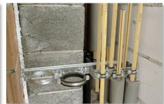
Pipe clamps and a variety of fittings can be installed easily on the hole matrix by standard threaded rod or screws.
