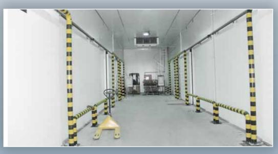
Depending on the size and use of the cold room, cold rooms can be broadly classified as walk-in cold rooms and warehouse cold stores. Cold rooms are built by TSSC to maintain a temperature range of 15°C to -40°C. Walk-in cold rooms are smaller in size compared to the large warehouse cold stores and are used primarily by the retail industry to store goods with fast shelf replenishment rate.
