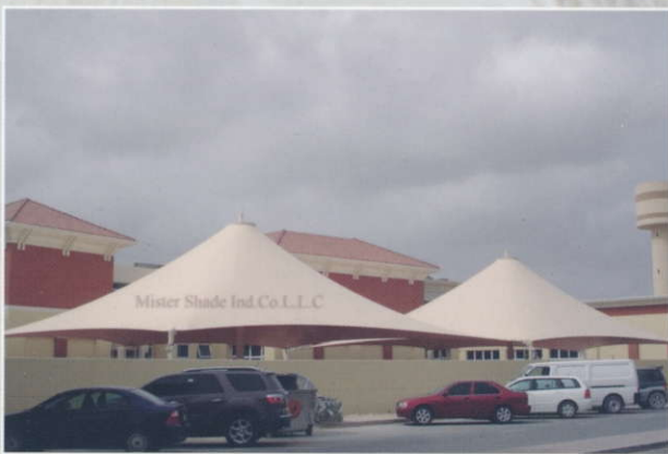
Assembly Shade in Rashidiya School - Dubai
